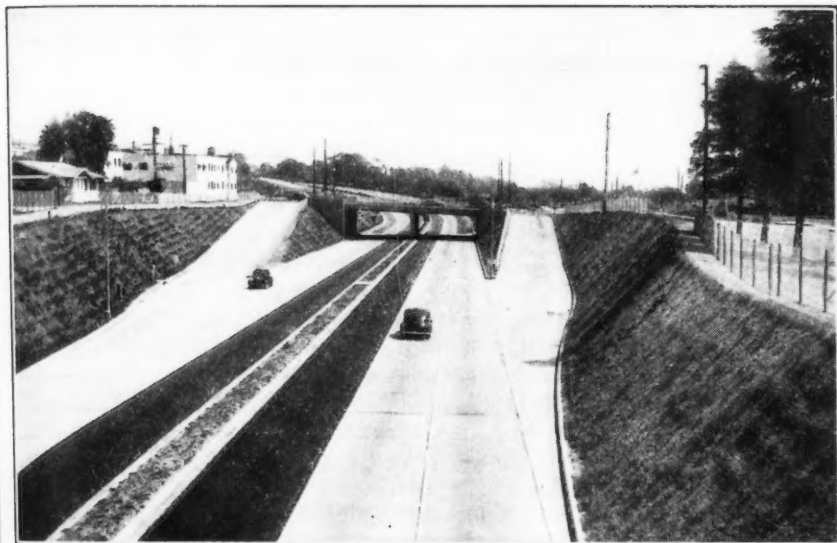
FIG. 14.—THE ARROYO SECO PARKWAY AT FAIR OAKS AVENUE, SHOWING TYPICAL ENTRANCE AND EXIT RAMPs OF COMPRESSED CLOVER-LEAF DESIGN
